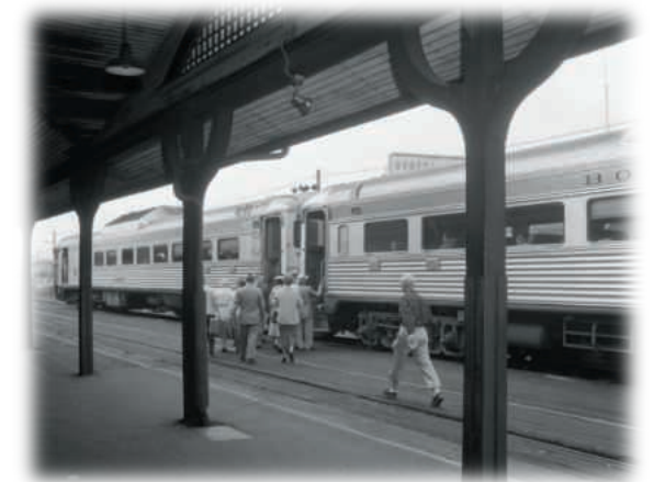
Passengers boarding a train at the Boston & Maine Railroad Station, 1958
