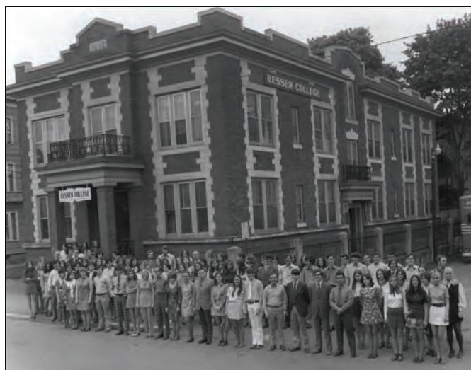
Photograph, Hesser College students in front of the college building, 155 Concord St. Manchester, June 1971 Donated by Mount Washington College/Hesser College
